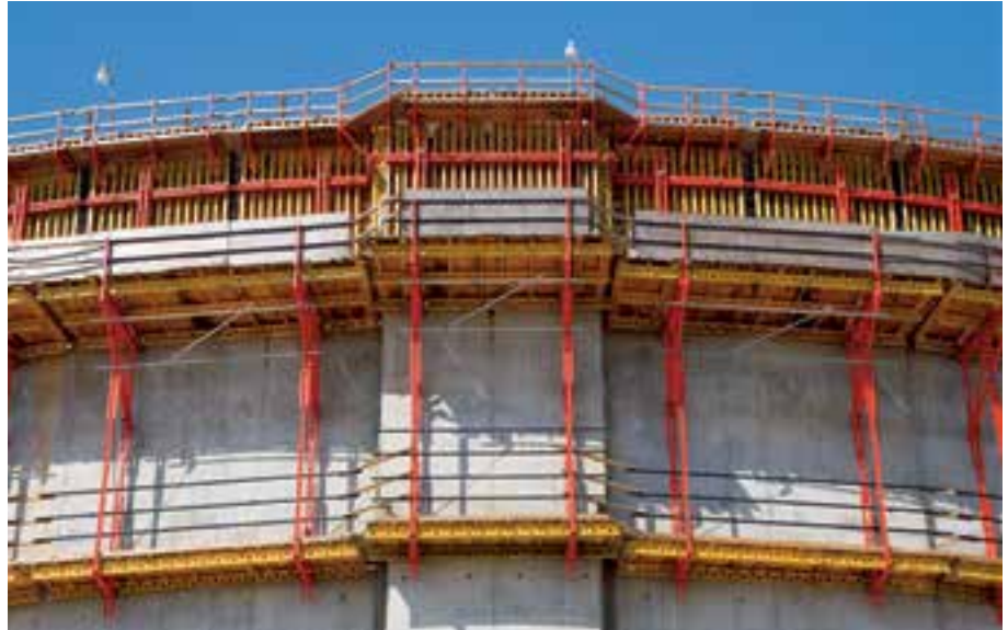
CB 240 Formwork carriage in working position Formwork carriage in concreting position
