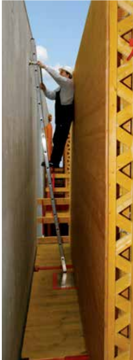
Safe working conditions on the CB 240 in protection of the formwork element.
