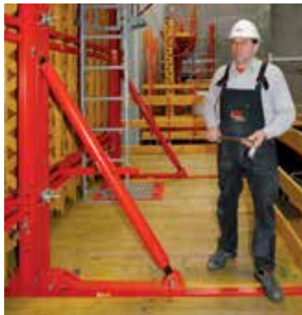
Safe and secure movement on the CB 240 working platform.
