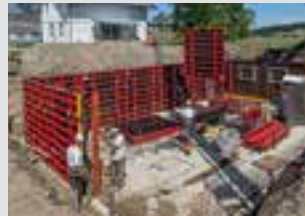
Wall Formwork
