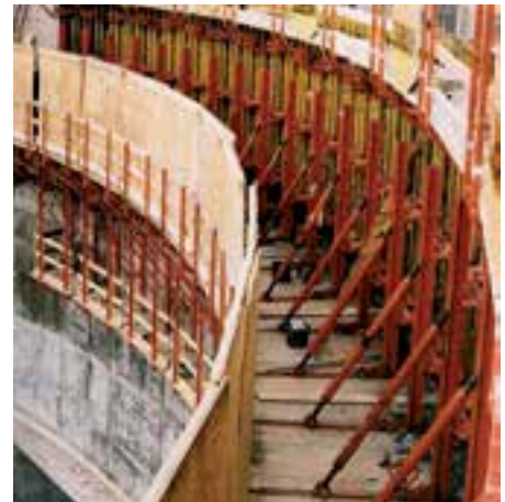
Closed platform decking for safe working.
