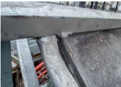
Access Deck UAL ■ defective welding seam on the mounting
