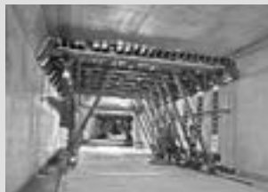
Tunnel Formwork
