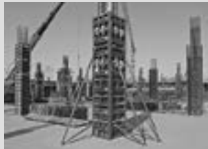
Column Formwork
