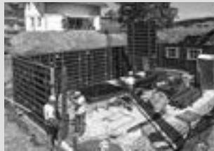
Wall Formwork
