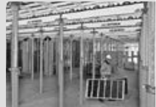
Slab Formwork
