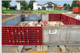
Wall Formwork
