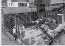
Wall Formwork
